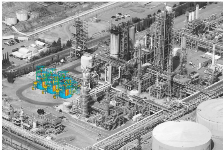
Figure 3: The Hazer Process has a similar footprint but fewer inputs than SMR
