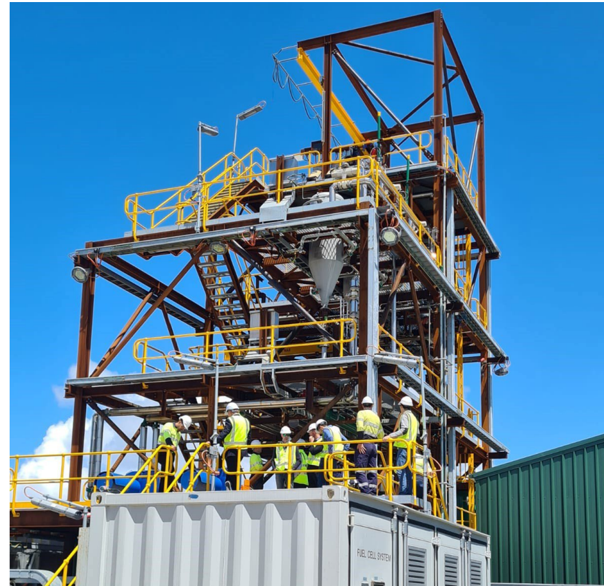
Suncor & Fortis CDP Site Visit - October 2022
