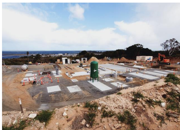
CDP Construction Site at 2 September 2021
