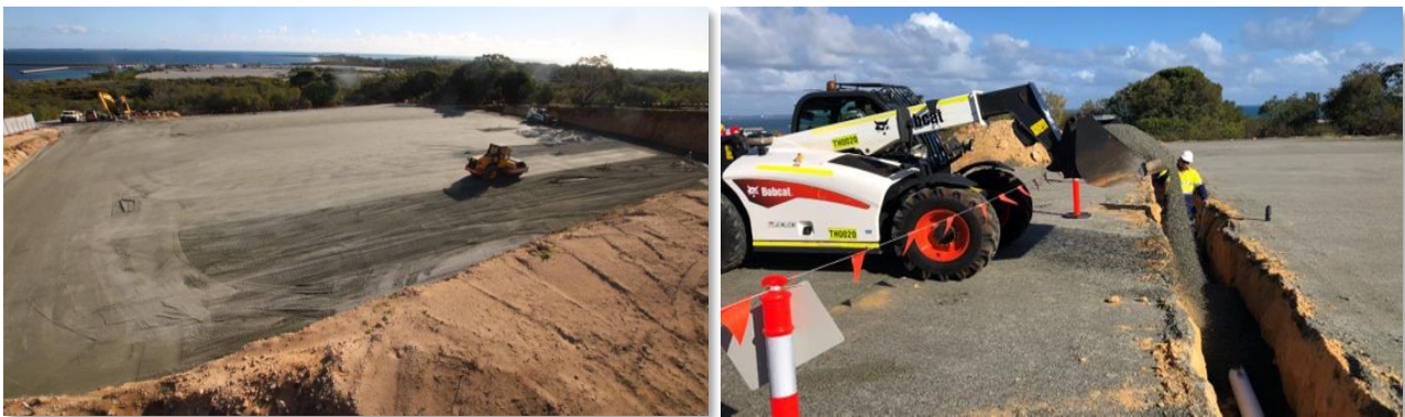
Site compaction & laying foundations
