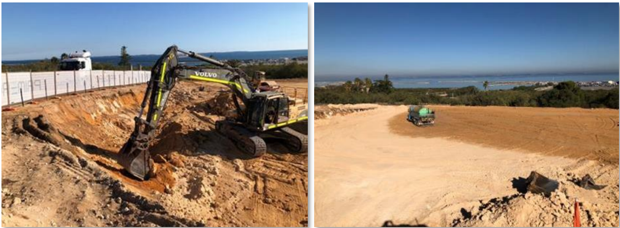
Commercial Demonstration Plant – site preparation
