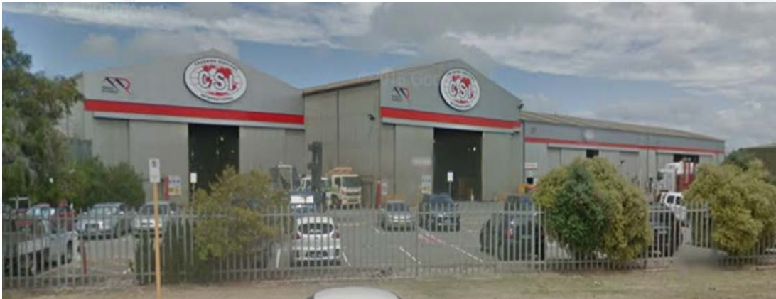
Photo: MRL site for the new pilot plant located in Kwinana, Perth.
